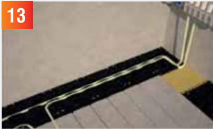
13 Complete the first circuit and connect the return pipe to the manifold using a euro cone connection. Repeat all circuits.
