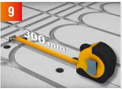
Additional use of ProWarm<sup>™</sup> screws and washers is recommended over timber substrates where needed, fixed at every 300mm.
