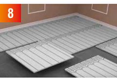
Bed the boards, primed side down, into the adhesive and ensure compression of adhesive ridges, ensure full compression of the adhesive to give a void free full adhesive bed.
