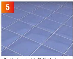
Grout the tiles using UltraTile Flex Joint grout. Allow to fully cure before trafficking.
