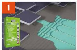
Fix the tiles using UltraTile ProFlex S2 adhesive. Ensure that every pipe channel and void surrounding the pipe is fully encapsulated with tile adhesive.
