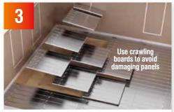
Lay the boards across the floor with the grooves facing upwards, making sure the pipework runs are calculated correctly to reach manifold position.
